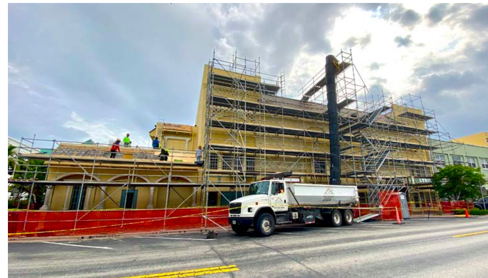
2021 With amazing community support for The Next Act Capital Campaign, The Lyric underwent critical structural and building renovations including substantial structural column and beam replacement/repairs, new roof, new air conditioning units and restoration of the marquees.
