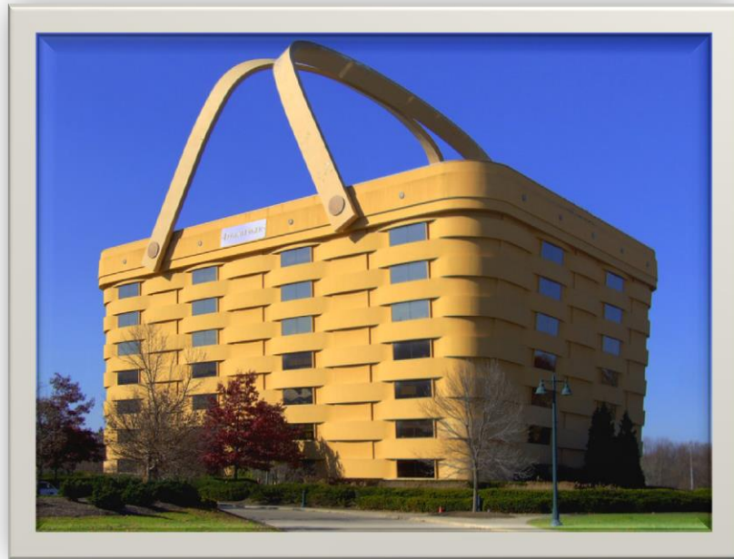
Above: No, this isn't a lawn ornament or a picnic for a giant! This building is the corporate headquarters for the Longaberger Basket Company located in Newark, Ohio. Inside this basket are seven stories of offices where great ideas happen every day!
